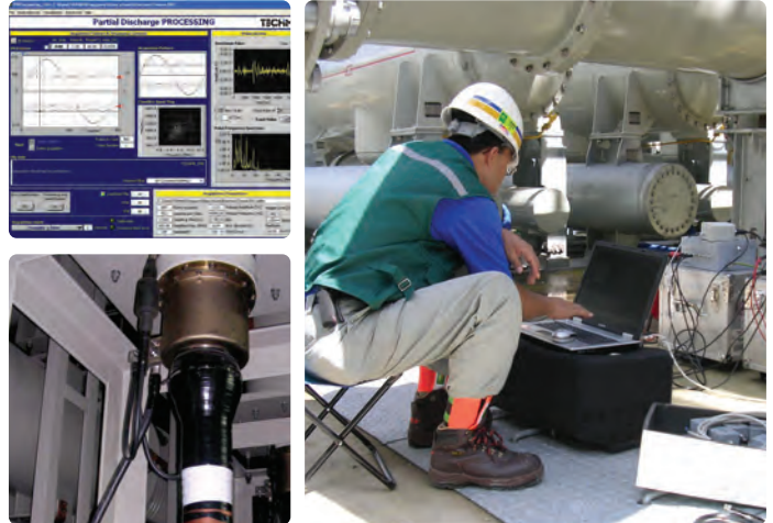
(2) On-site PD Detection on EHV Cable (Termination)
